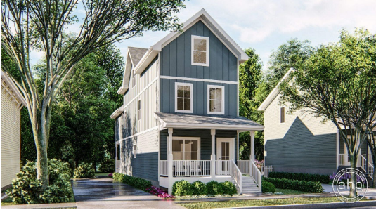
GARAGE ENTRANCE IN REAR
